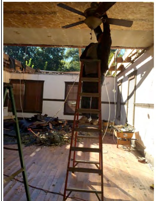
A recent photo of the meeting room shows the roof & ceiling damages.
